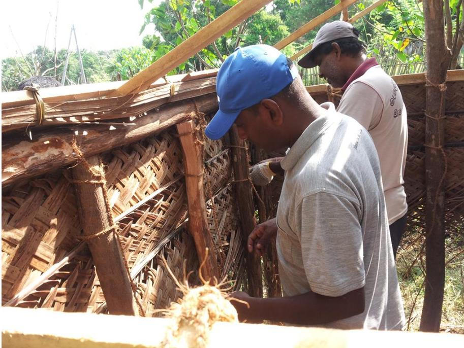
Figure 3. Horizontal arrangement of cajdan
